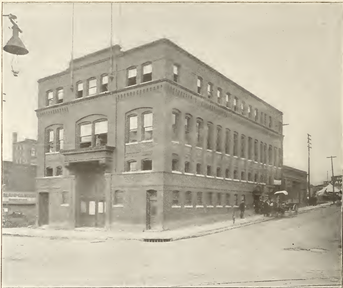
Divisional Headquarters, Hall and Metzpole, Kansas City, Mo.
